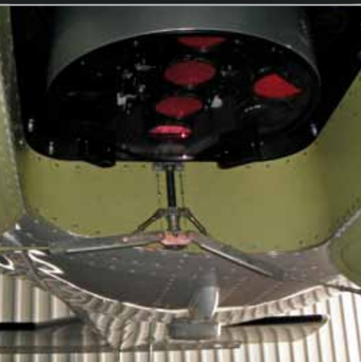
Installation in Vulcanair P68 View from floor hatch
